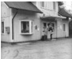
Kårsta station (se_ab_tahf_4230)
