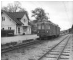
Kårsta station (se_ab_tahf_4231)
